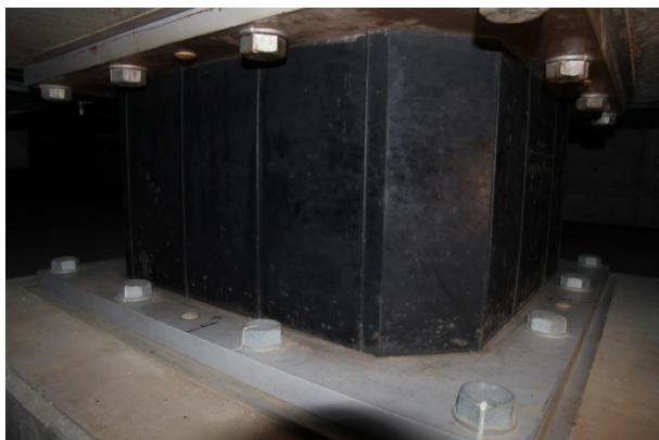
Figuur 2 detail base insulation oplegging
