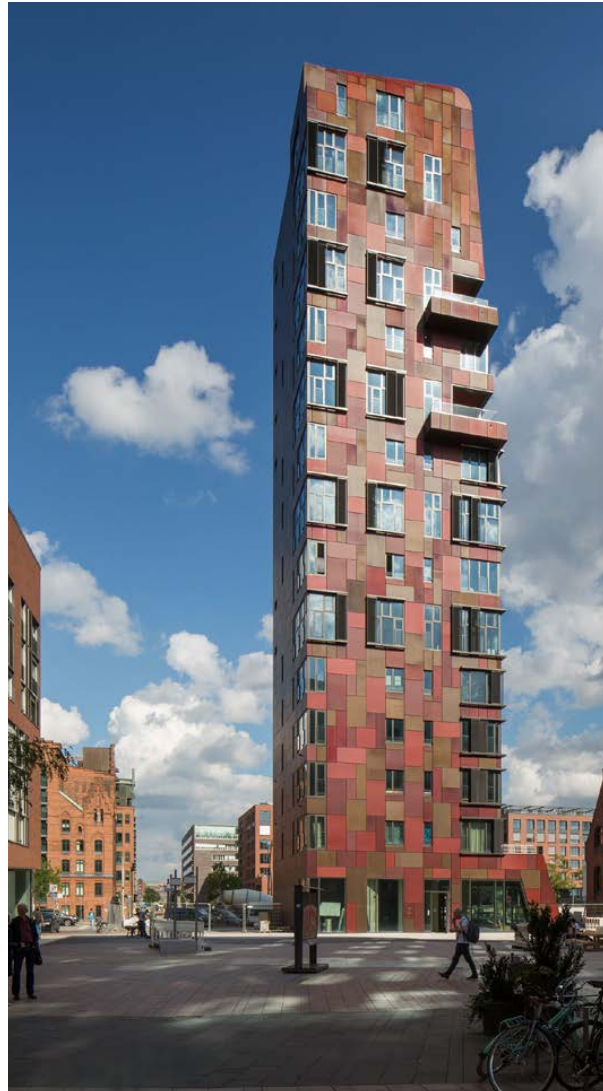
slanke toren. Cinnamon - Hamburg; architect: Bolles+Wilson
