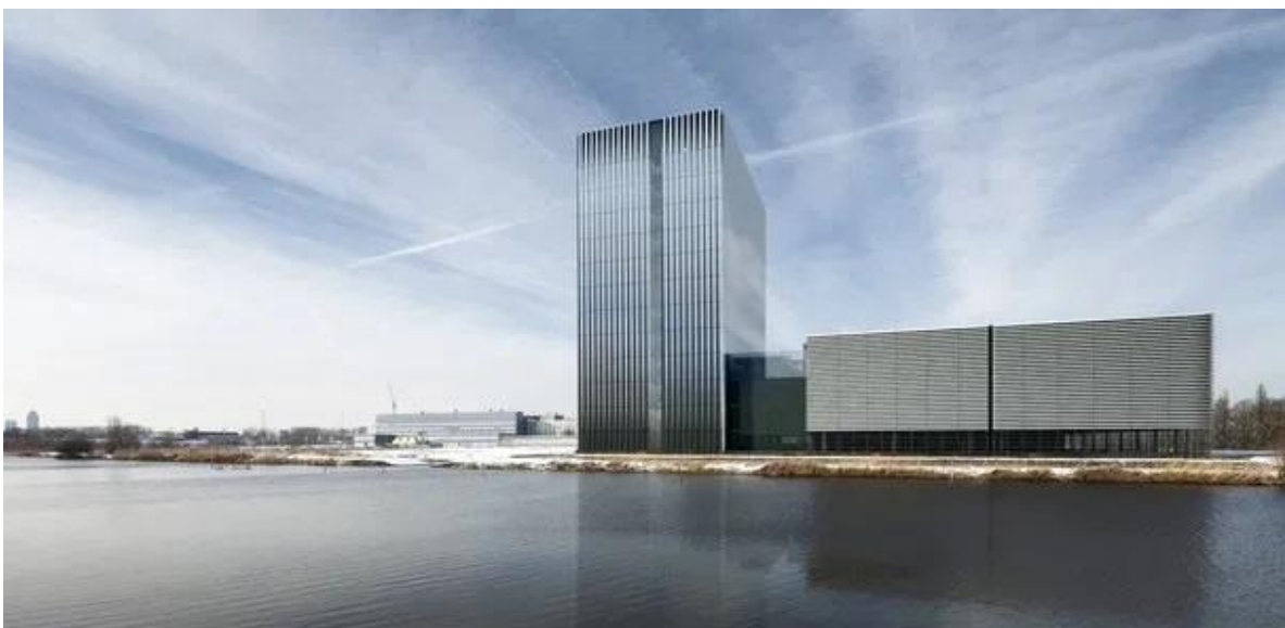
AM4, Equinix datacentre, 2014-17, by Benthem Crouwel Architectss ©Jannes Linders
